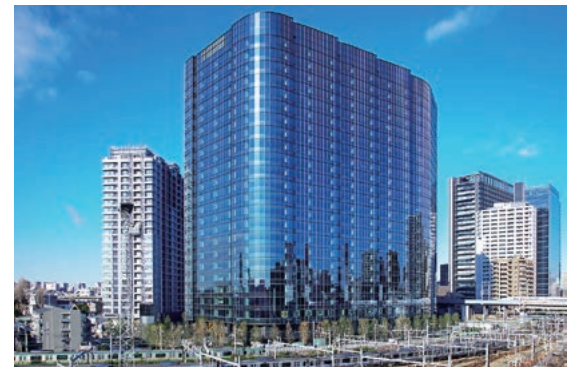
Head Office Building (Osaki)
