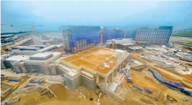
Construction site at the end of July 2016
